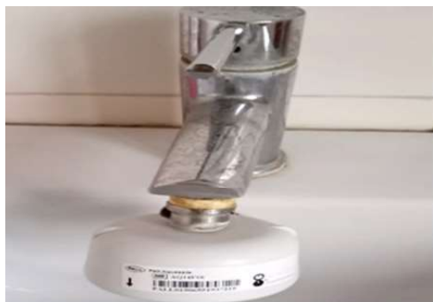
Fig. 6: Pall Aquasafe Water filters installation
