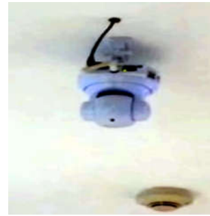
Fig. 1: Wall mounted IP camera
